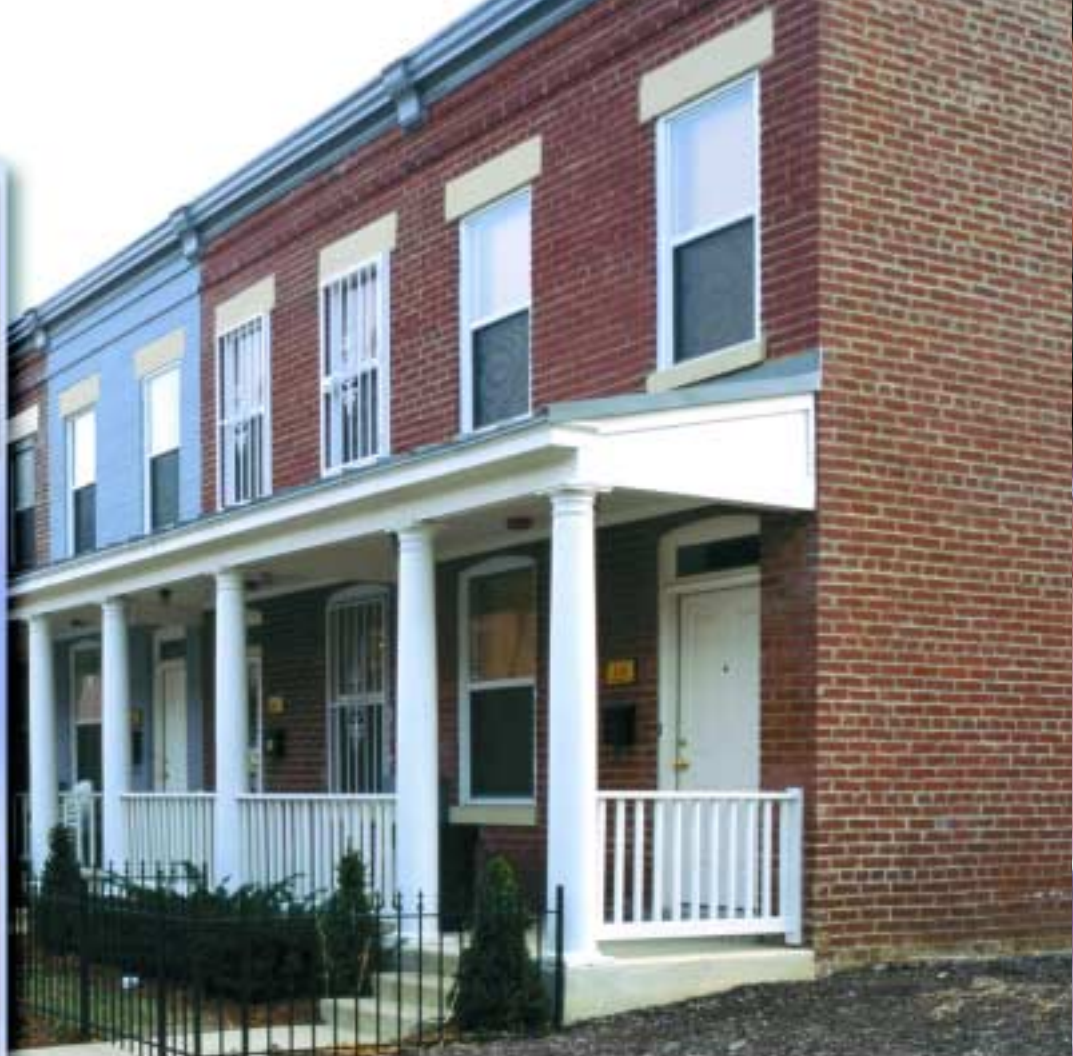
With commitment and extensive planning by Howard and Fannie Mae, new LeDroit Park residents (left) are beginning to enjoy the vitality that has been restored to the neighborhood.
